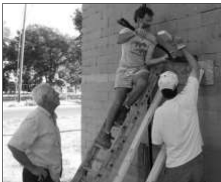
Eric Shankland and Doug Woodworth repair a hole in the grange
