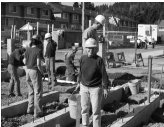
Marcia Gordon and crew prepare the townhome foundation
